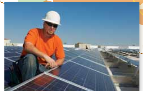
Southwestern alignment takes advantage of abundant solar energy potential.
