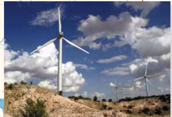
Eastern terminus sited to take advantage of abundant wind energy potential.
